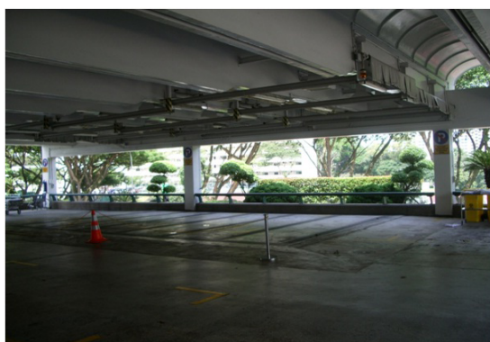
Figure 1A. Ambulance Parking Bay Immediately Outside the Department of Emergency Medicine (DEM) Entrances
